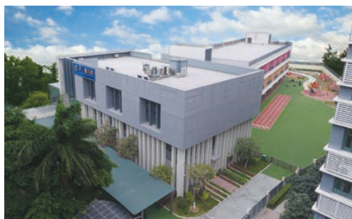
2016 - ELFA Foshan, Guangdong Province
